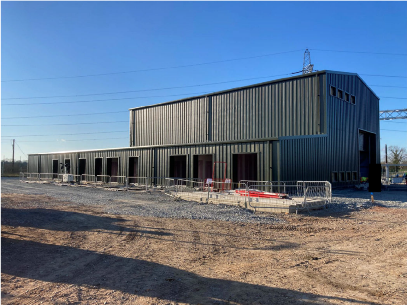
Image 3.8 Existing National Grid 400 kV Substation at Yaxley (Source: National Grid)
