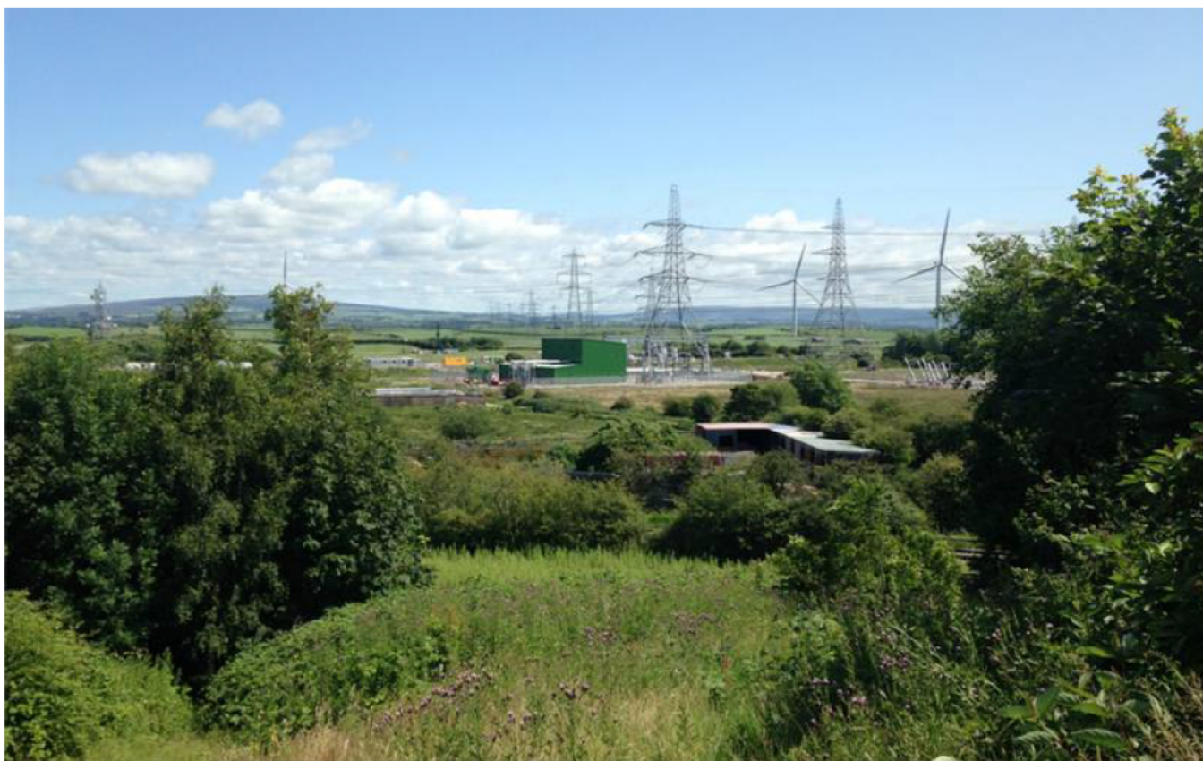
Image 3.5 Existing Middleton 400 kV Substation (Source: National Grid)
